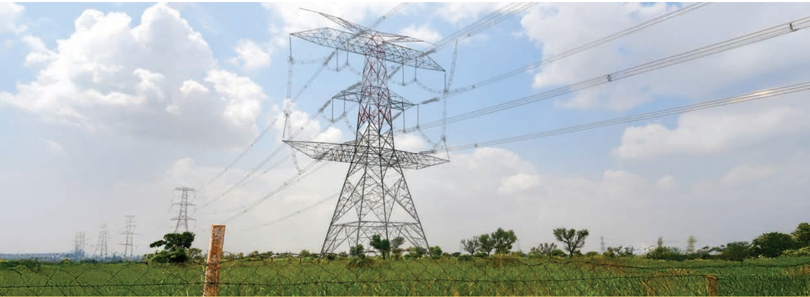
A Transposition Tower along the 765 kV Fatehgarh–Bhadla Transmission Line in Rajasthan
