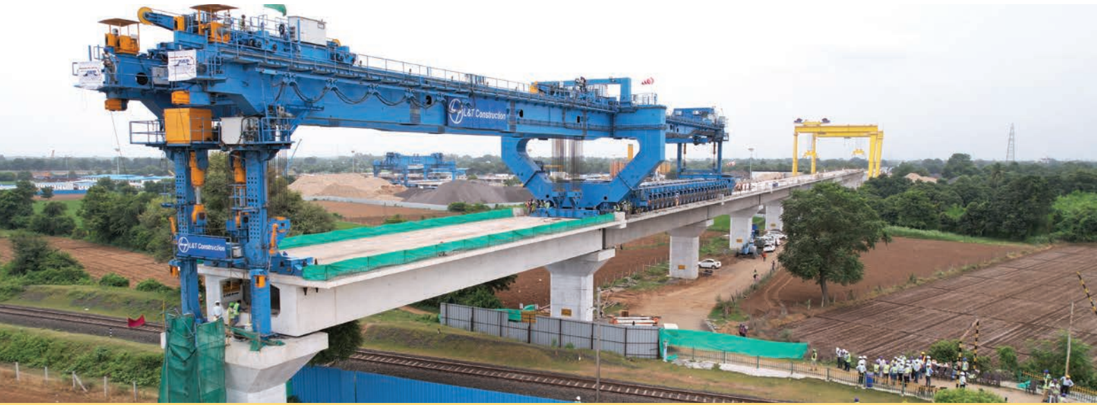
Launching Girder manufactured by Minerals & Metals - Product Business Unit, in action at the High-Speed Rail Project in Anand, Gujarat
